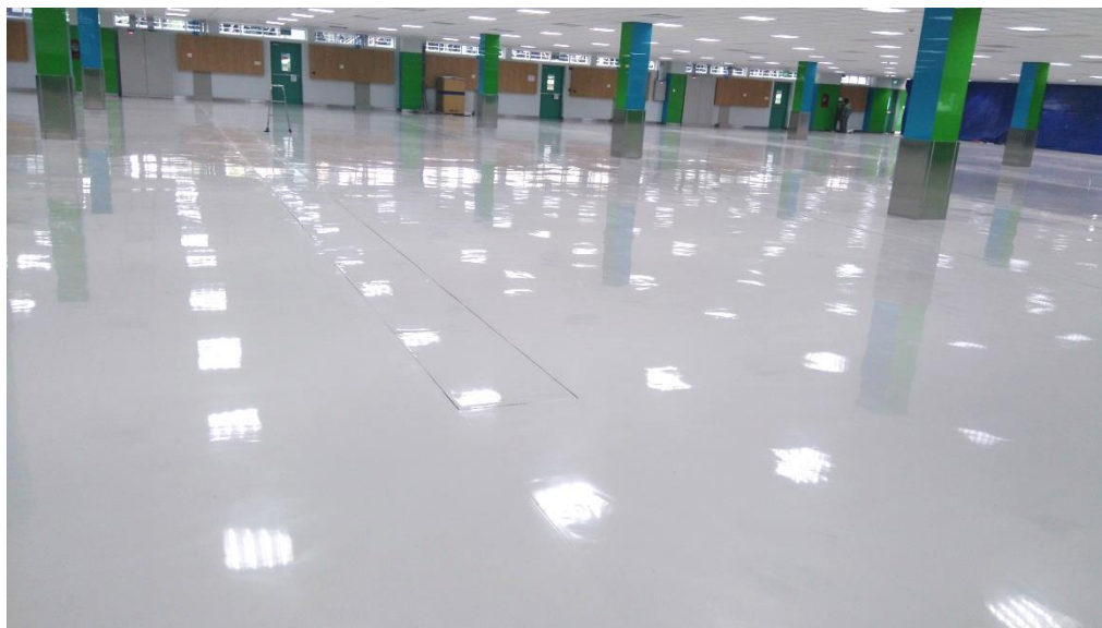
Picture: Sikafloor®-263 was applied on floor of Phonak factory
