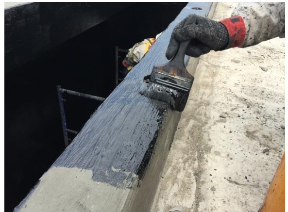
Picture: Sika® Poxita F was applied at Outspan Coffee Factory
