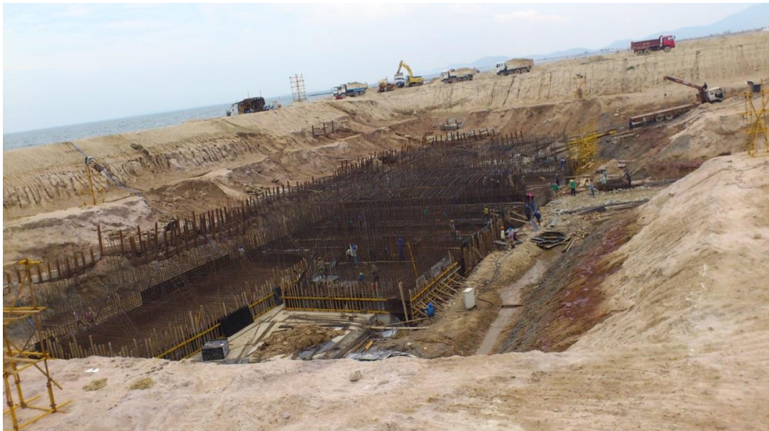
Picture: The treatment system for sea water into fresh water
