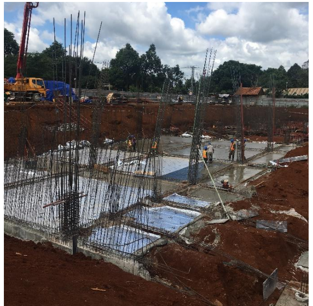
Picture: SikaBit® W-15 was applied on the floor retaining wall
