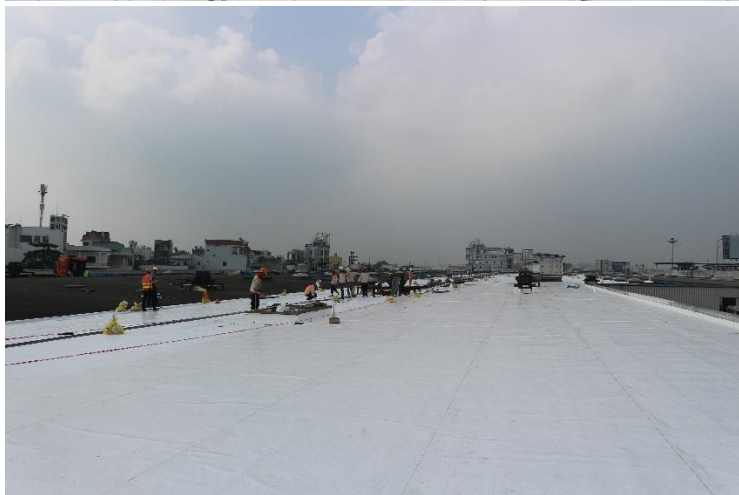
Picture: Application process of Sarnafil® S327-12L
