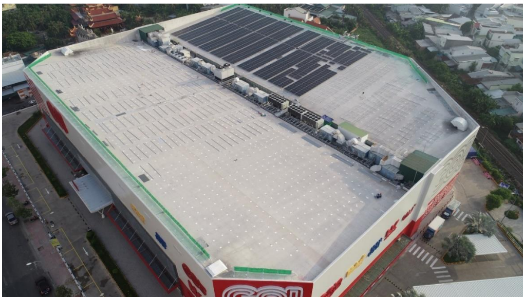
Picture: Sika Roofing system was applying on the roof
