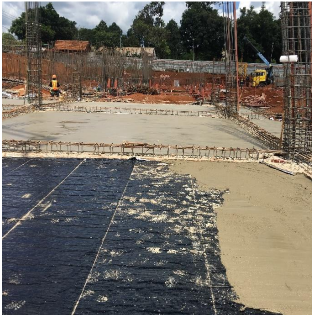
Picture: SikaBit® W-15 was applied on the floor retaining wall
