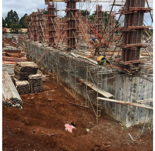
Picture: SikaBit® W-15 was applied on the floor retaining wall
