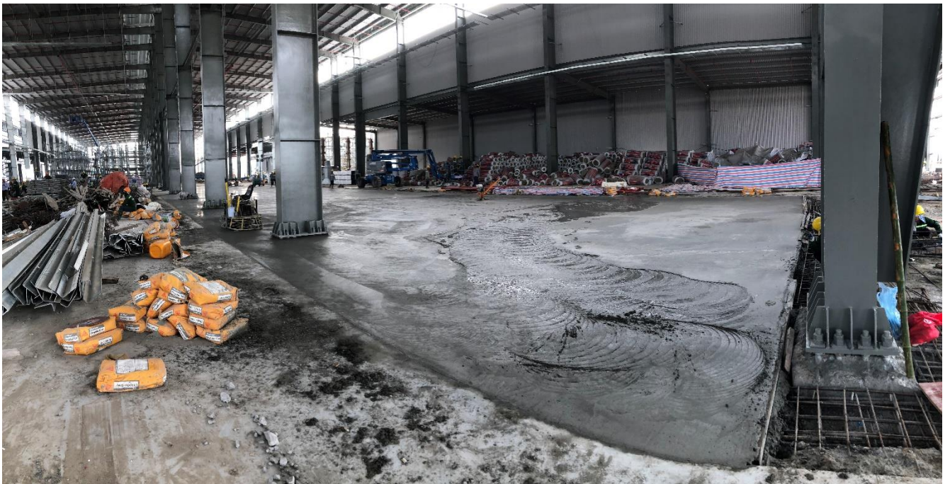
Sikafloor was applied at Vinfast project
