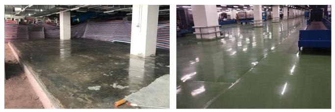
Epoxy self-levelling system Sikafloor®-263 SL HC at baggage sorting areas
