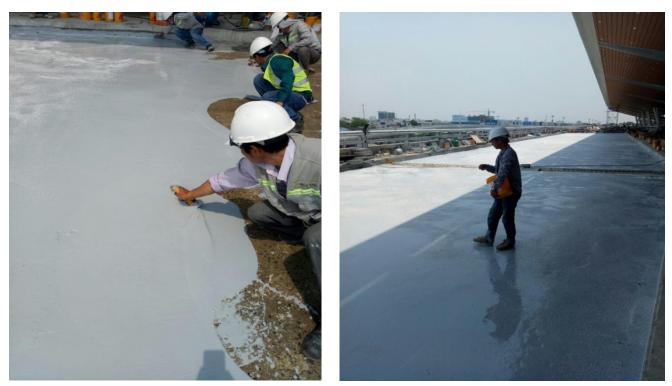
Sikalastic<sup>®</sup>-8326 system at overpass bridge deck
