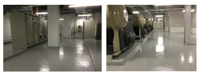
Epoxy coating system Sikafloor®-264 HC at technical room
