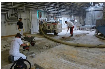
**FRIDAY AFTERNOON:** Mechanical removal of old tiles and epoxy adhesive. Substrate preparation and cleaning.
