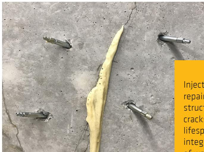
Injection of cracks is a common method used to repair and waterproof cracks in existing concrete structures. It can permanently seal even the smallest cracks and voids, contributing to enhance the lifespan of the structure, to recover the structural integrity of the concrete and to avoid the entrance of water, moisture or air through the crack.
