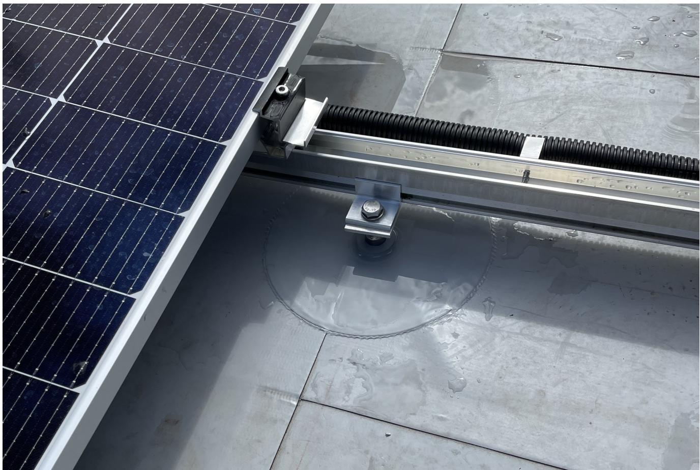
**SikaRoof® Anchor-W PVC** is a manufactured preformed accessory providing a secure watertight connection directly between the roof substructure/roof deck and waterproofing membrane.
