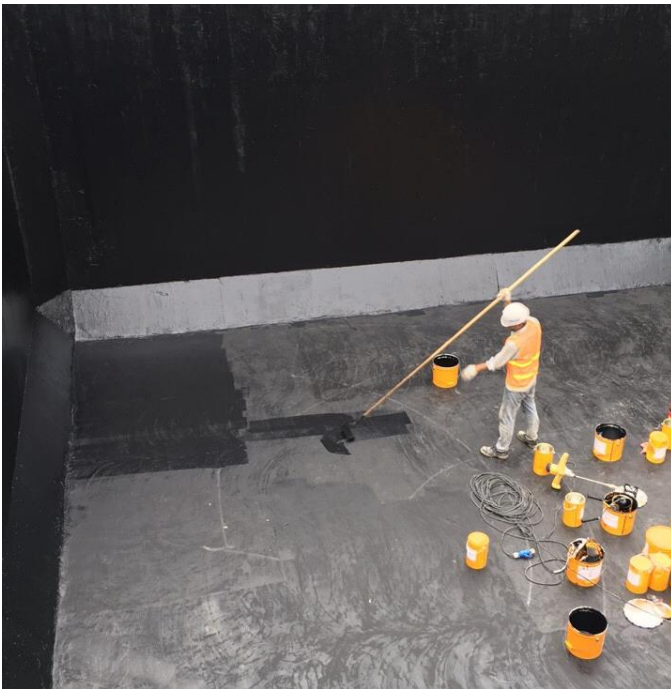
Picture: Sikafloor®-81 EpoCem® New HC was applied at Nestle Bong Sen with system of Sikafloor®-81 EpoCem, Sika® Poxita F
