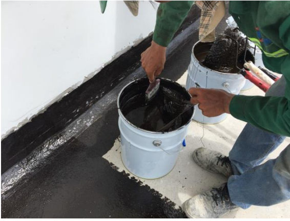
Application of primer, 1 st coat and 2 nd coat Sikalastic®-680 AP by brush or roller
