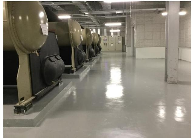
*Epoxy coating system Sikafloor®-264 HC at technical room*
