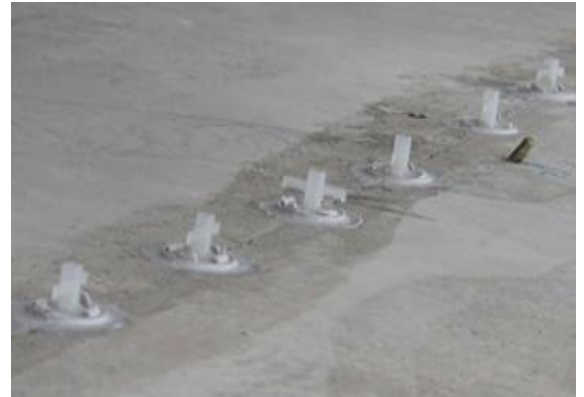
Sealing cracks by Sikadur®-731 and fixing plastic bowls onto crack lines
