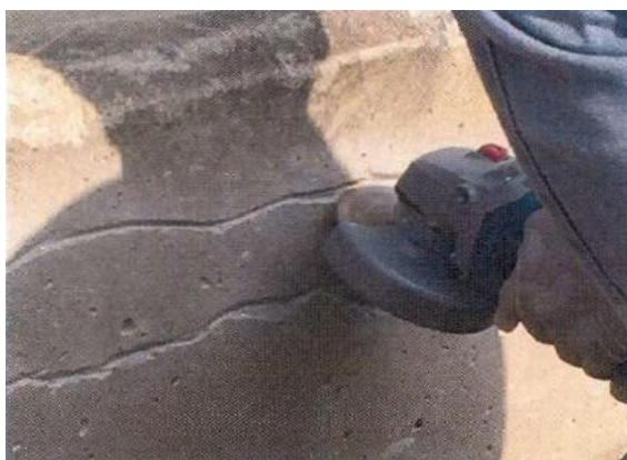
Grinding along crack line
