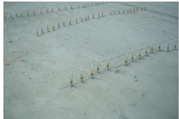
Fixing of cylinders and injection of Sikadur®-752
