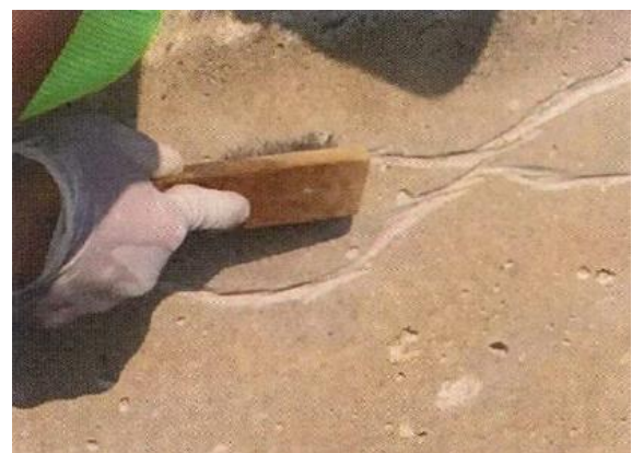
Cleaning crack line by steel brush
