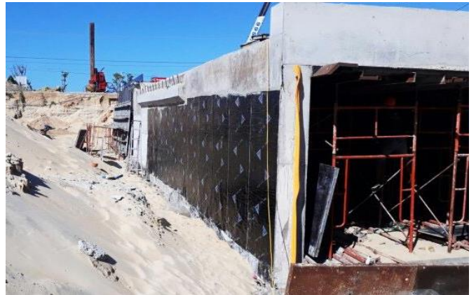
Picture: SikaBit® W-15 was applied at Surpass Tunnel_Mongomerie Link Golf Course project
