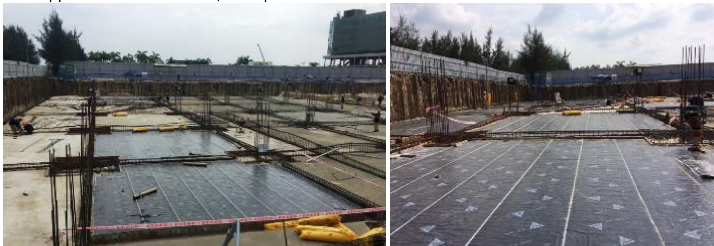
Picture: SikaBit® W-15 was applied at Cocobay project
