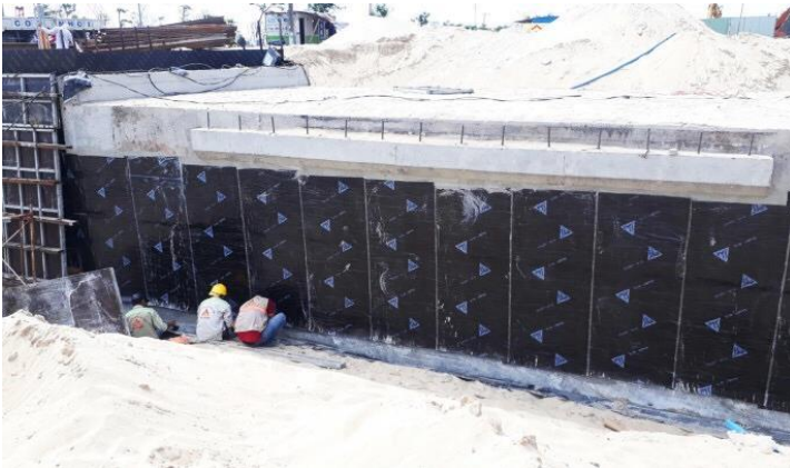
Picture: SikaBit® W-15 was applied at Surpass Tunnel_Mongomerie Link Golf Course project
