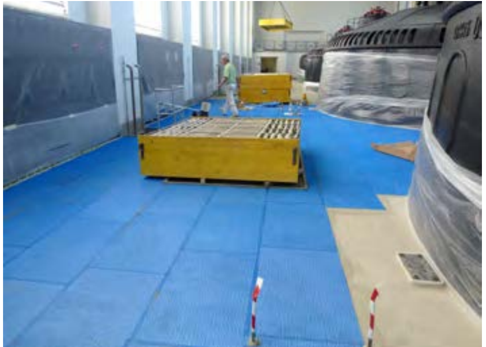
The decoupling mat Sika® Permat is being installed.
