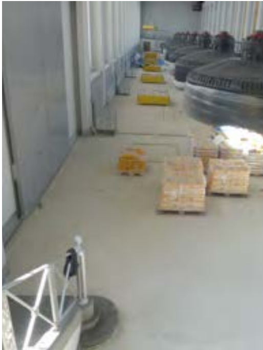
The levelling layer was ready 24 hours later.
