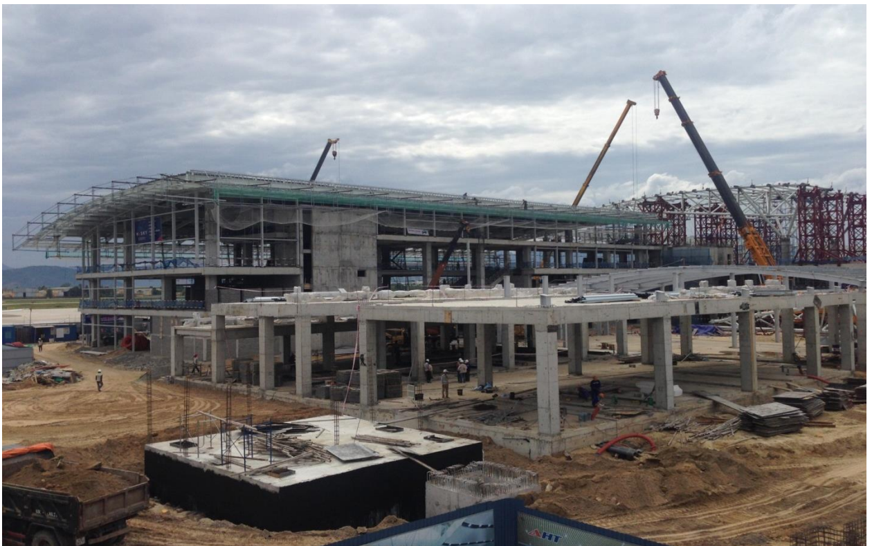
Picture: Sikaproof® Membrane was applied in Terminal 2 of Da Nang Internation Airport project
