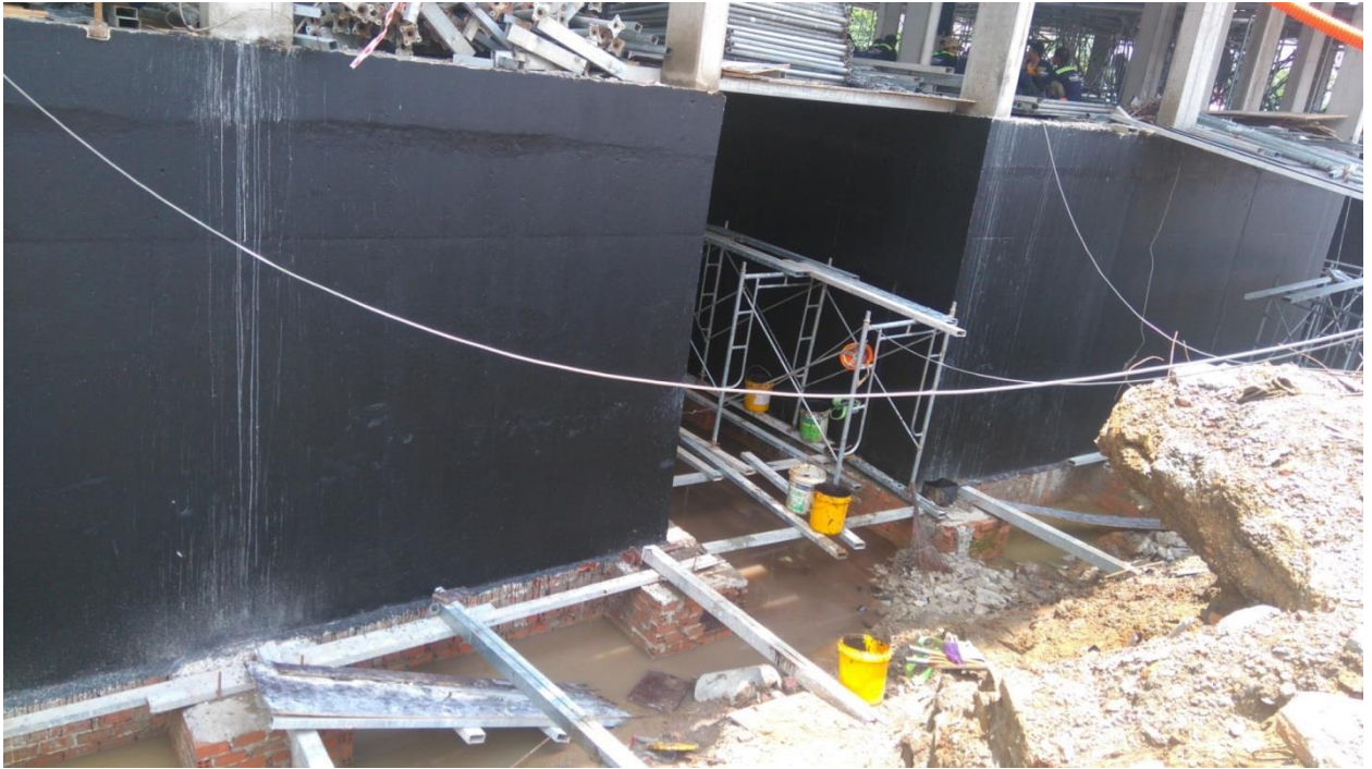
Picture: Sikaproof® Membrane was applied in Vinhome Golden River project
